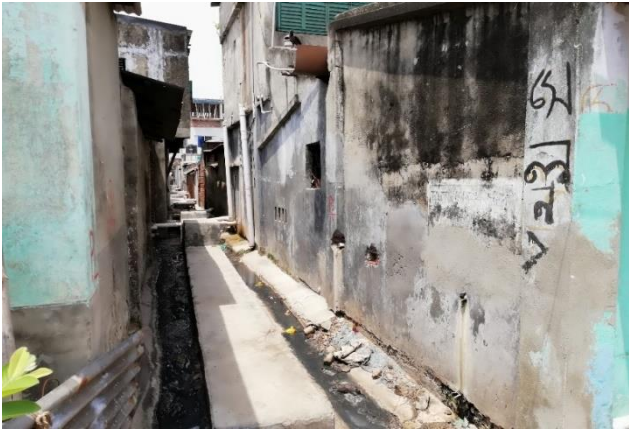
Figure 5 Post-intervene site situation.
